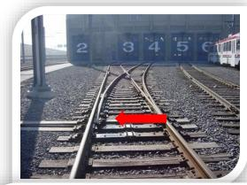
Facing Movement: The movement of a train over a switch whose points face in the direction opposite to which the train is moving.
