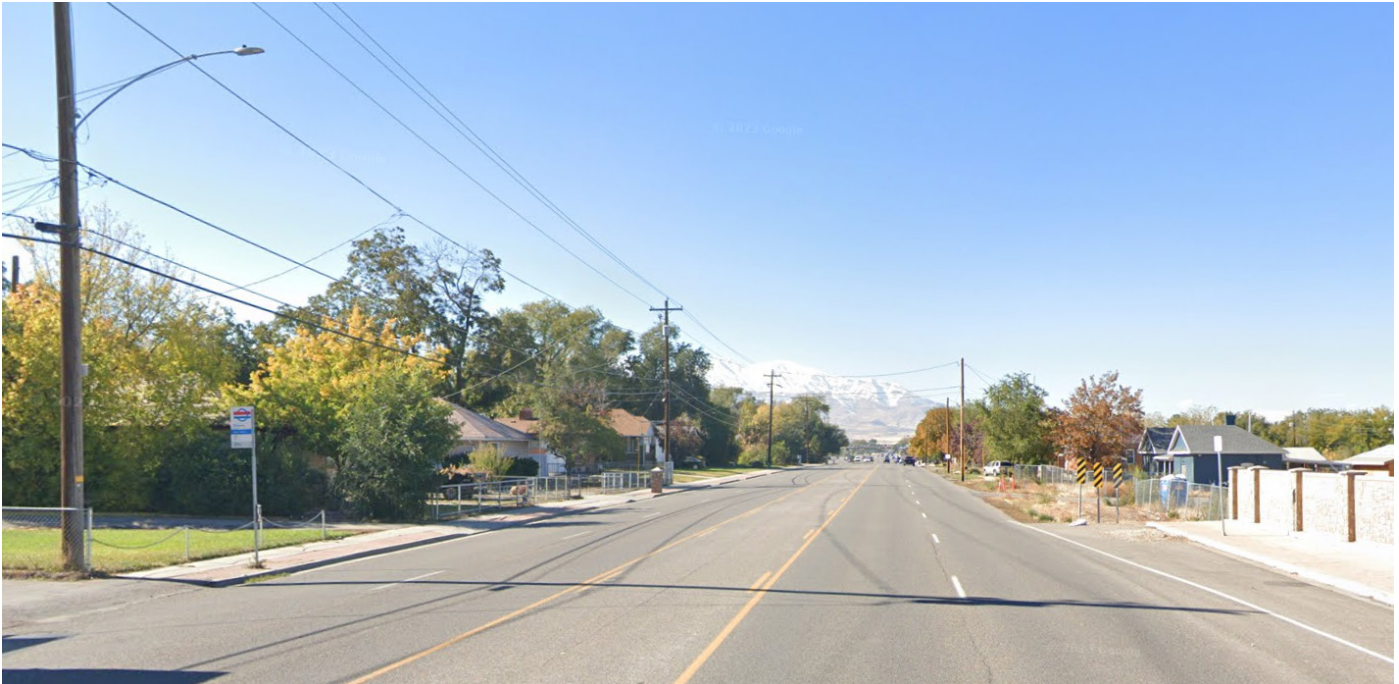
Figure 2. An incomplete sidewalk and limited access to basic transit and active transportation infrastructure along this section of 3500 South, in an Equity Focus Area in West Valley City, highlights the need for equity in transit and active transportation planning.
